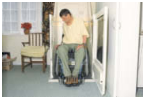
Figure 10.5 A complete C6 tetraplegic patient using a through-floor lift at home.
